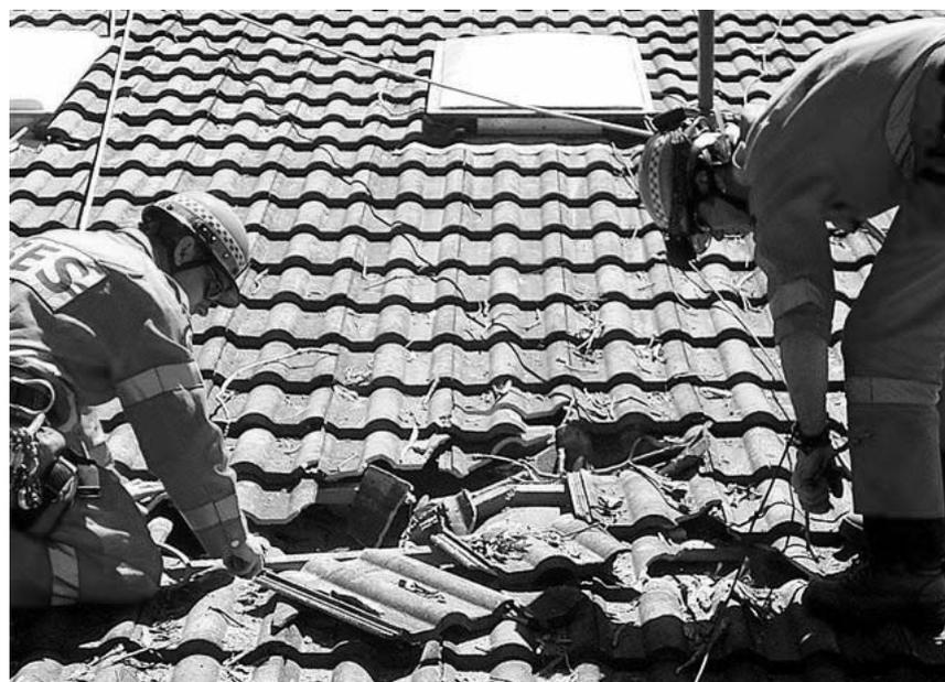
SES volunteers providing emergency repairs to the storm-damaged roof of a home in Sydney's eastern suburbs following a hailstorm in April 1999
